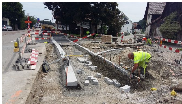
Abb. 3: Randabschlüsse alte Seonerstrasse
